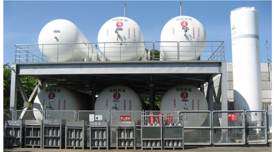
Warm storage vessels at Taiwan's National Synchrotron Radiation Research Center
